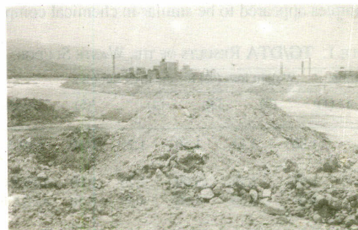
Fig. 2. A part of the disposal site area covered with the thick deposited PAF waste.
